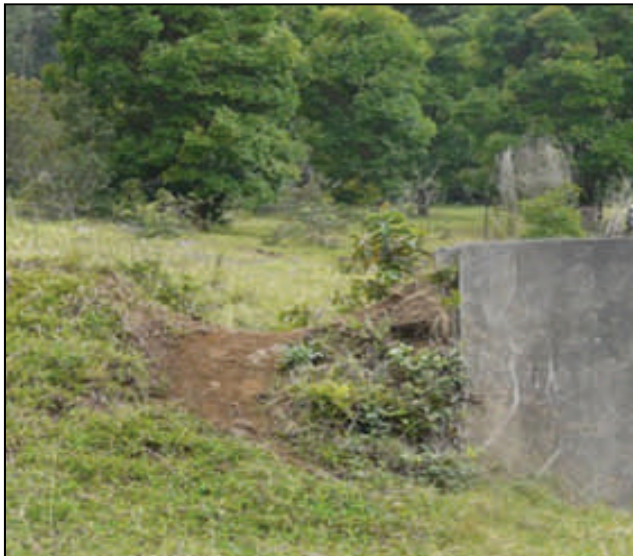
The animal trail in the above picture has affected the integrity of this flood control structure .
