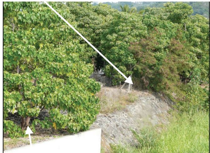
Kukui nut tree whose root growth can create problems in the future with the integrity of the concrete wall.
