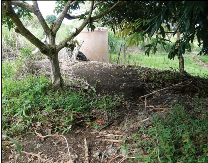
Sediment built up along a fence line. It might look like extremely fertile soil but it came at the cost of the fence.
