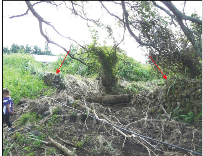
Prior to the 5/6 rainfall there had been a complete rock wall between the two red arrows.
