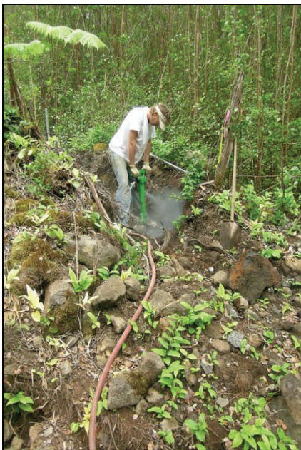
Far left: Using a jack hammer to install fence posts in pahoehoe. Top center: more holes for fence posts. Bottom center: Fence posts complete, moving on. Far right: completed fence, now for the restoration.
