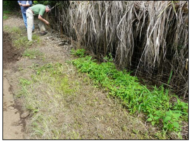
Description: GPS point 329, where the county used to access a flood control structure. Due to a fence and extensive christmasberry growth they are no longer able to do so. They plan to dig out some of this so that water can flow more easily into the sediment basin area from the road instead of traveling down the road.
