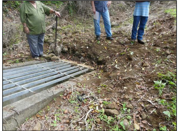
Description: Another shot of flood control structure KD-5. The shows the depth of sediment in front of the concrete lined pit. Normal sediment level should be approximately two feet below the inlet to the structure.
