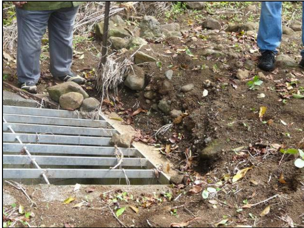
Description: Flood control structure #3 at GPS point 330. After the 5/6 storm event .large boulders were covering this grate.
